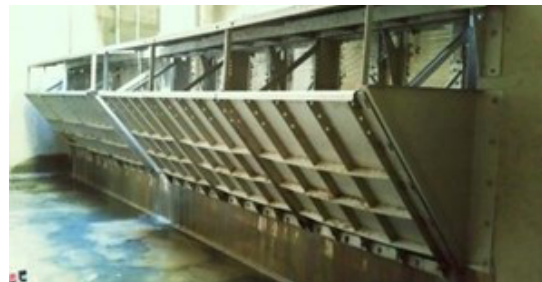
Figure 16: Vertical bar screen. Source/credit: Hydroconcept
