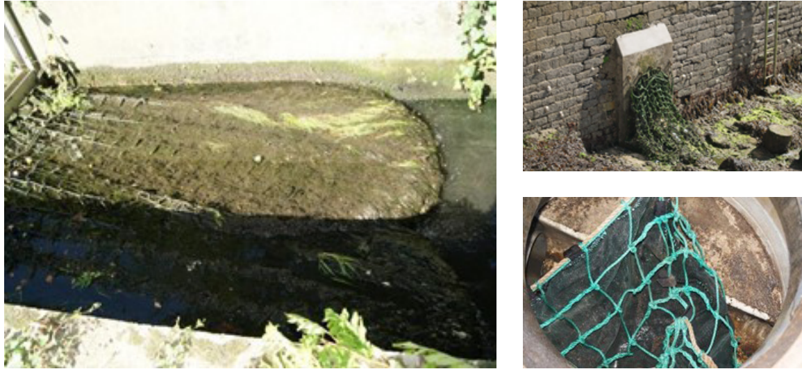
Figure 12: Retention nets in place in Brest Métropole in waterways, rainwater outlets and downspouts (Photos OiEau)
